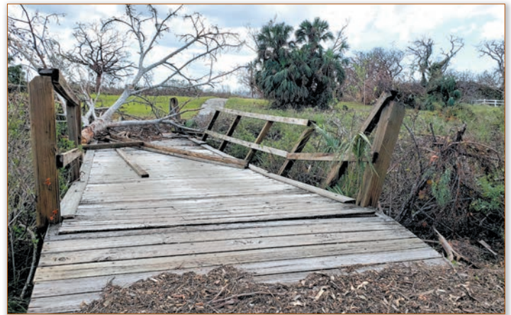
Canal Foot Bridge severely damaged by hurricane.
