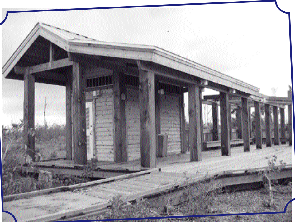
A direct hit from Hurricane Charley on our partially constructed public facility had virtually no effect. (Photo by J. Worth)
